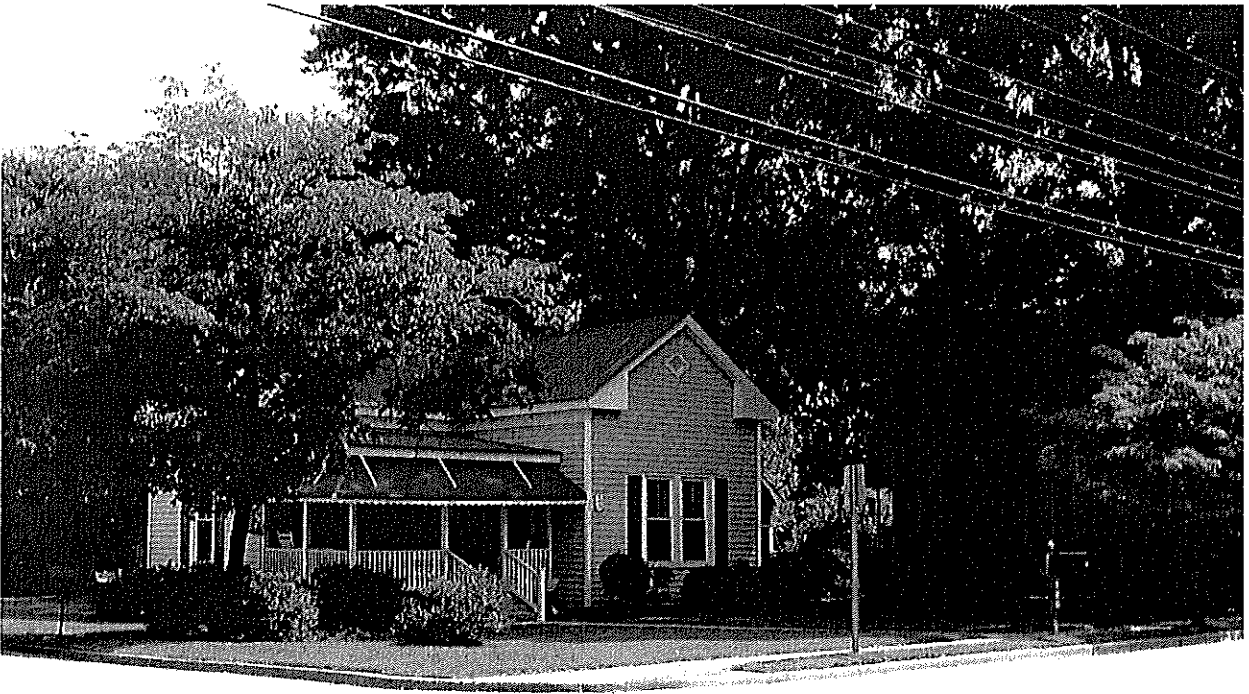
Property No. 1 – Brooks House (#120 W. Hargett Street). Main (south) and west elevations.
